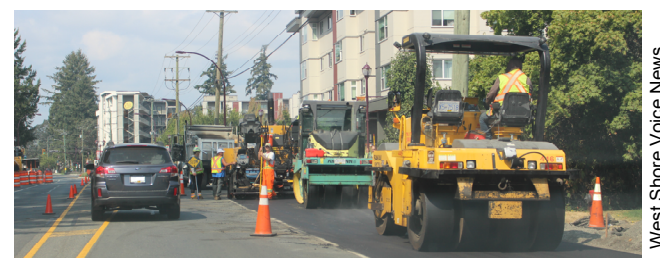
Paving on Goldstream Avenue (August 24).
