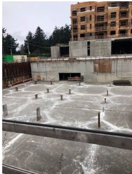
Construction at the Colwood Corners residential/commercial development this week.
