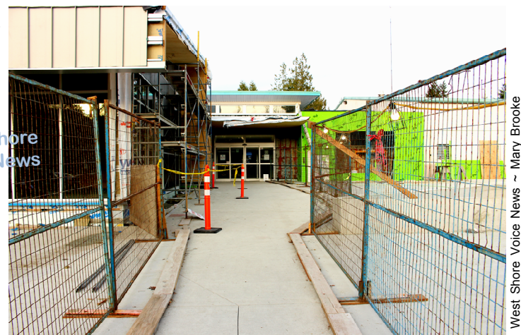
Expansion underway at SEAPARC in Sooke (November 6).
