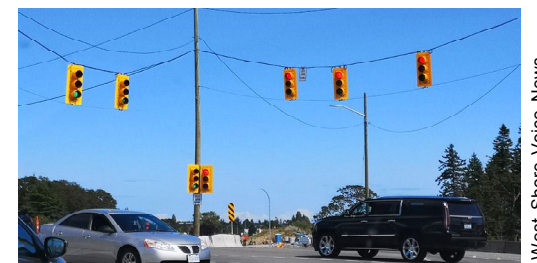
Temporary traffic lights Hwy 1 & McKenzie as restored after July 15 impact.
