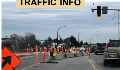
Langford Parkway roadworks near Westhills Stadium, March 6.
