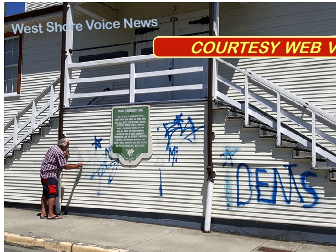
<< District of Sooke Councillor Rick Kasper was out at Sooke Community Hall on a hot summer Thursday afternoon, July 6, starting some of the graffiti removal from the front of the building.
