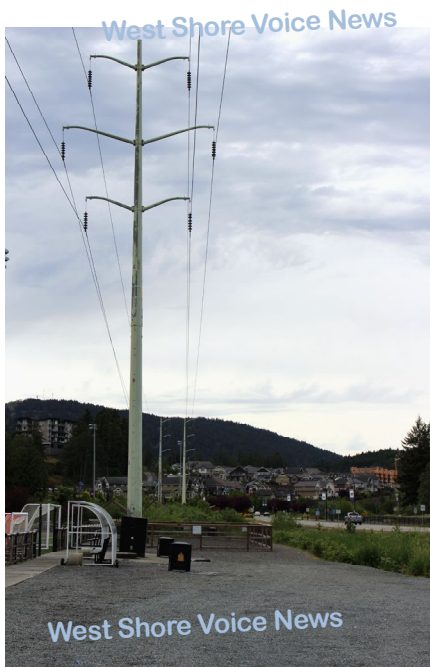
To put in a second set of bleachers at Westhills Stadium, this hydro pole carrying 230 kV transmission lines would need to be moved across the street.
