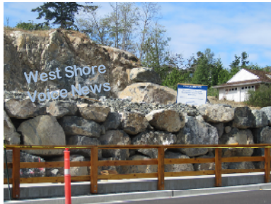
A retaining wall on Latoria Road.
